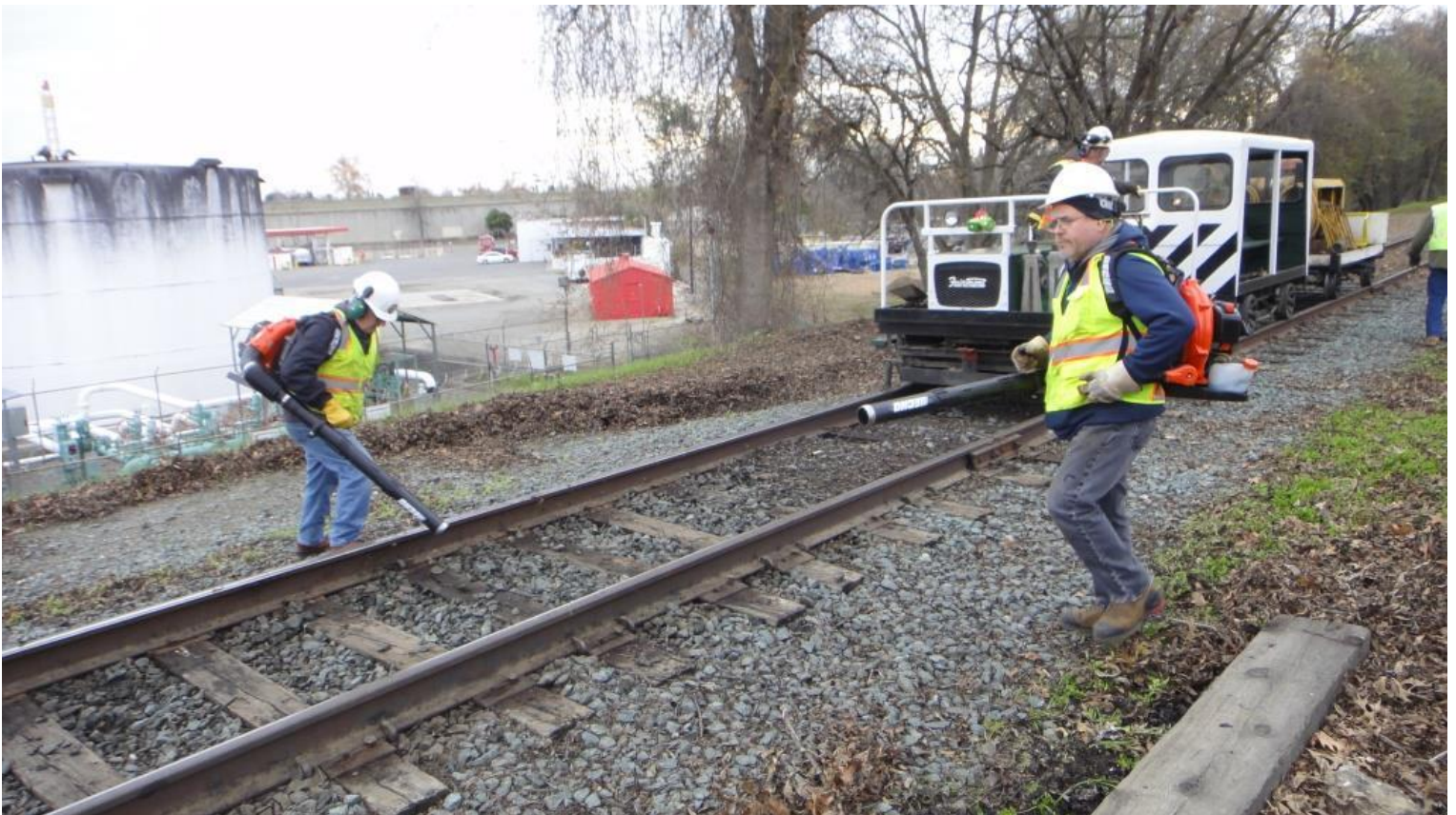
Mike W. and Steve W. don the huff-and-puff machines for the removal of organic debris from the SSRR Mainline at Oleander Alley
