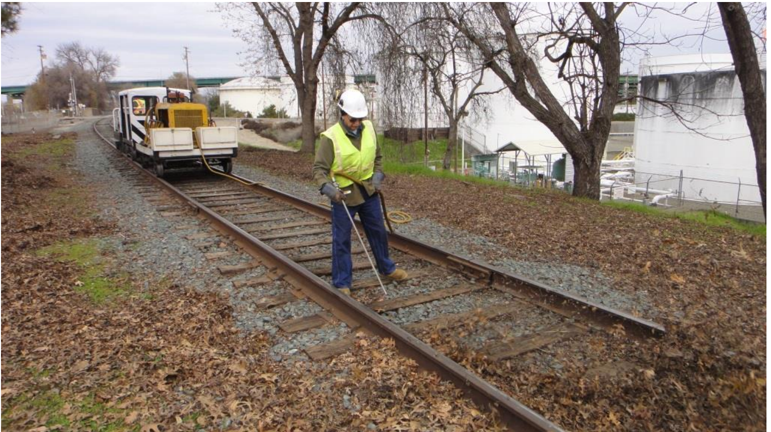
Once the compressor was working again, Clem took the air-wand out to spin-up some leaves
