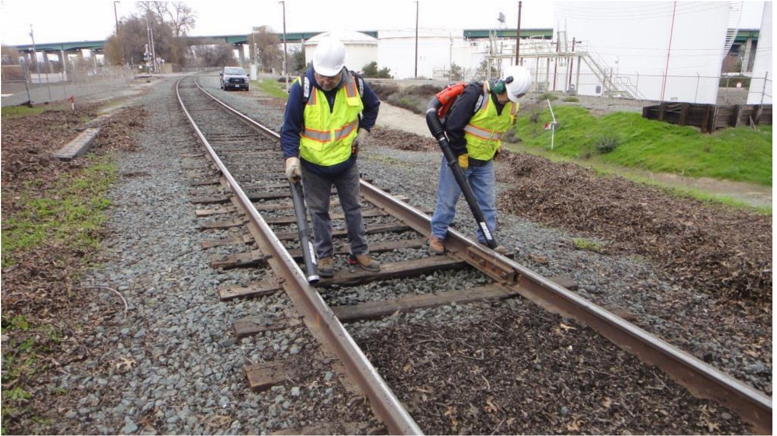
Steve W. and Mike W. did an amazing job clearing away mulch from the track
