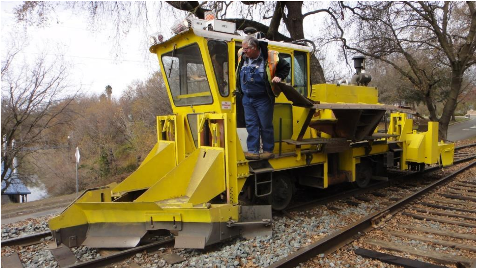
Chris guides the regulator as it plows and brooms the track
