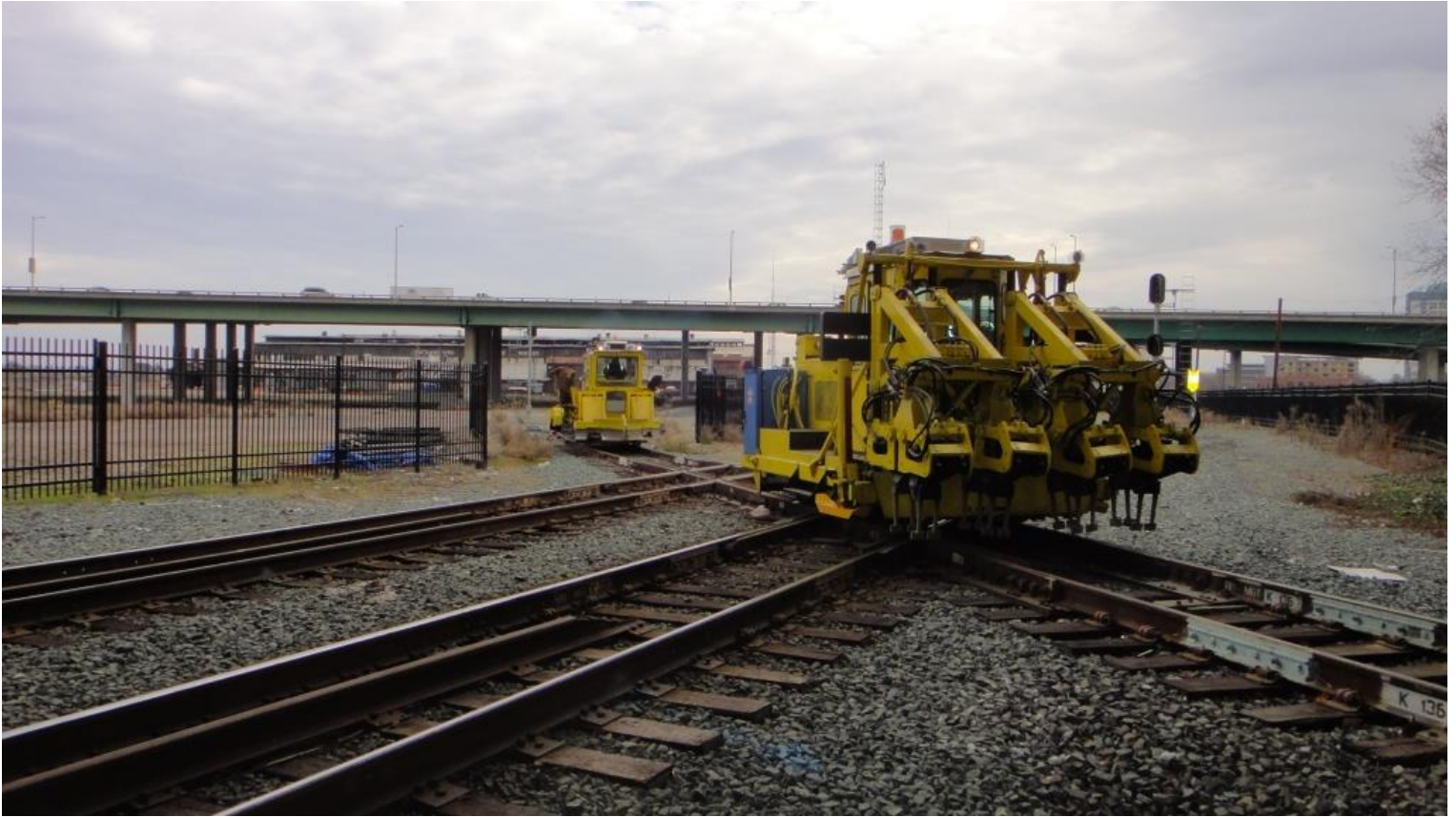
The mighty MOW tamper and ballast regulator crossing over the Union Pacific Mainline at RV-988
